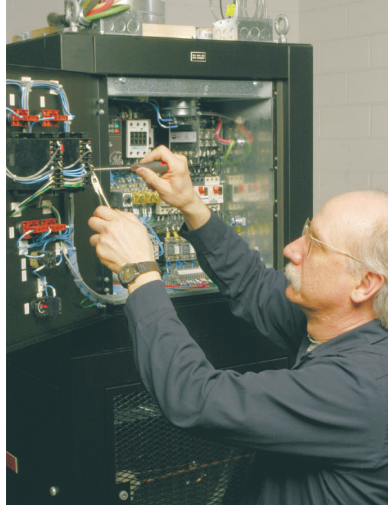
Jim Penfield makes final wiring connections on an AdvancAir unit.
