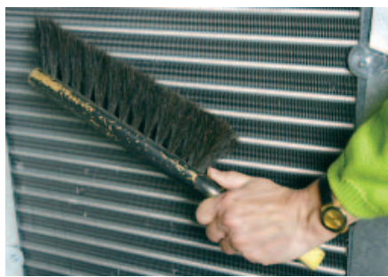
Regular cleaning of the condenser ensures a longer life for your cooler.
